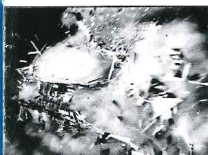
EFFECT OF NUCLEAR BLAST ON WOOD-FRAME HOUSE LOCATED THREE-FIFTHS OF A MILE FROM GROUND ZERO AT A NEVADA TEST SITE, 1953
